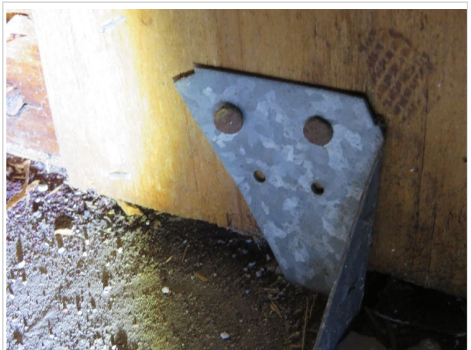
Roof to wall attachment clips
