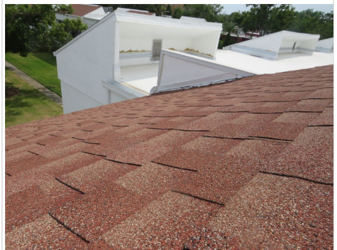
Roof covering asphalt shingles
